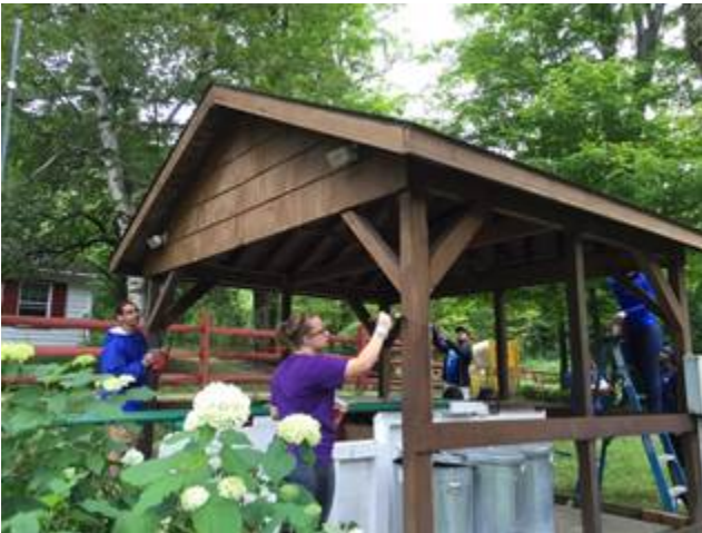
Volunteers apply stain to the pavilion at Highbrook Lodge
