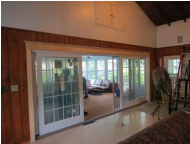
New sliding glass doors in Smith Lodge
