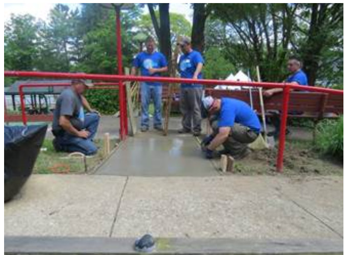
Volunteers measure the new concrete sidewalk
