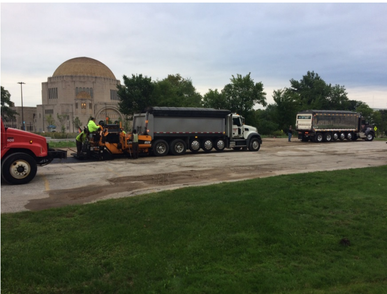
Trucks prepare the lot for new asphalt
