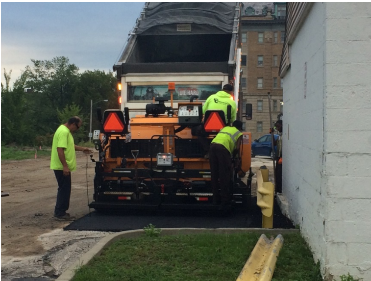
Workers lay new asphalt by the garage
