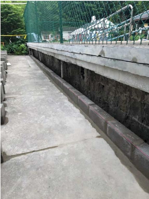
The new retaining wall along the pool at Highbrook Lodge
